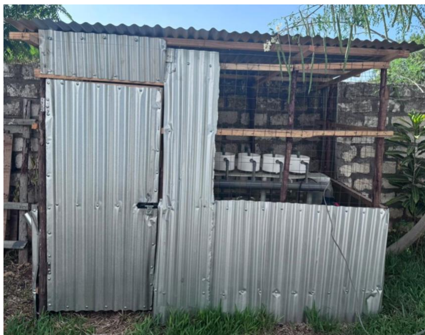
Figure 5: The newly constructed hatchery shelter to provide shade and security for the tilapia egg incubation unit. It helps prevent direct sunlight on the hatching jars which previously increased water temperatures leading to high egg mortality.
